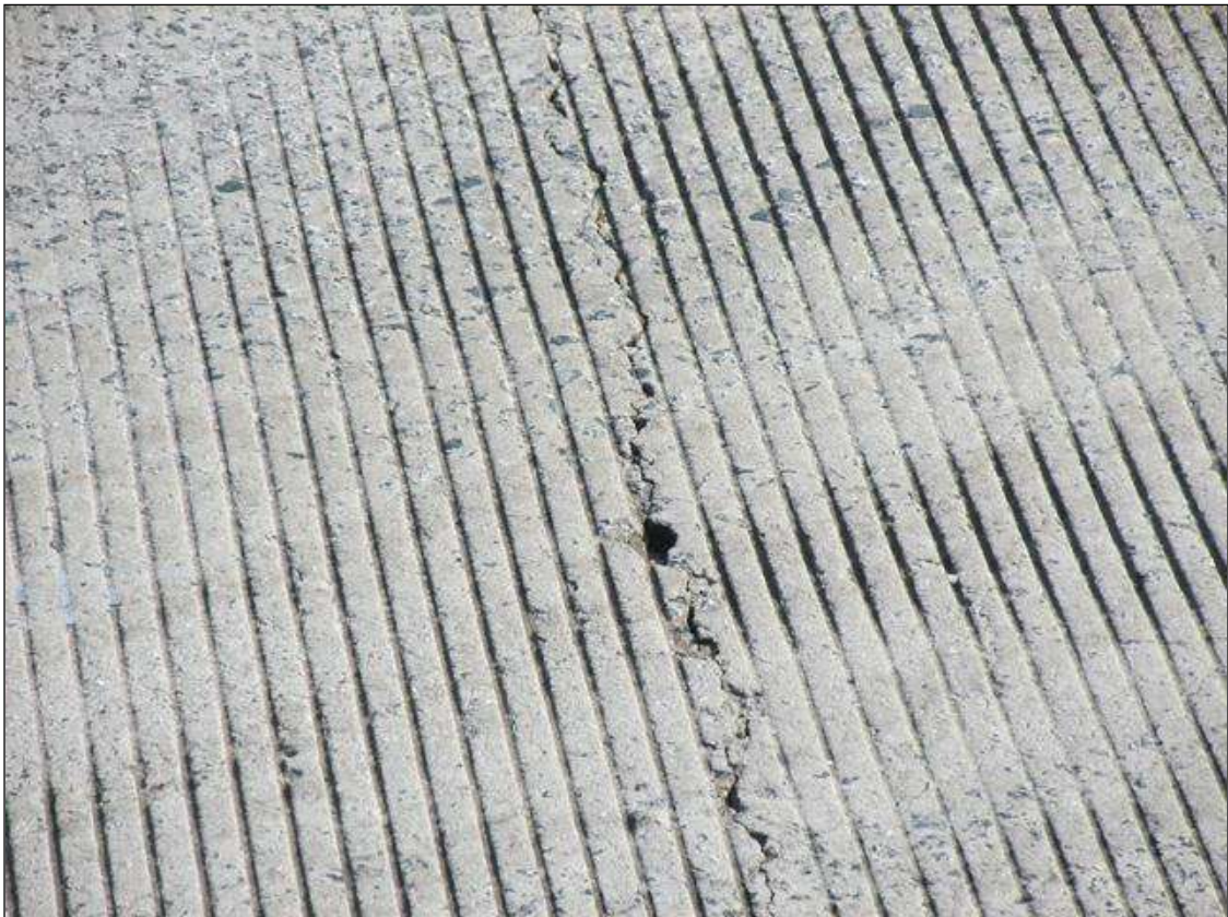
TRANSVERSE CRACKS IN ALL SPANS
