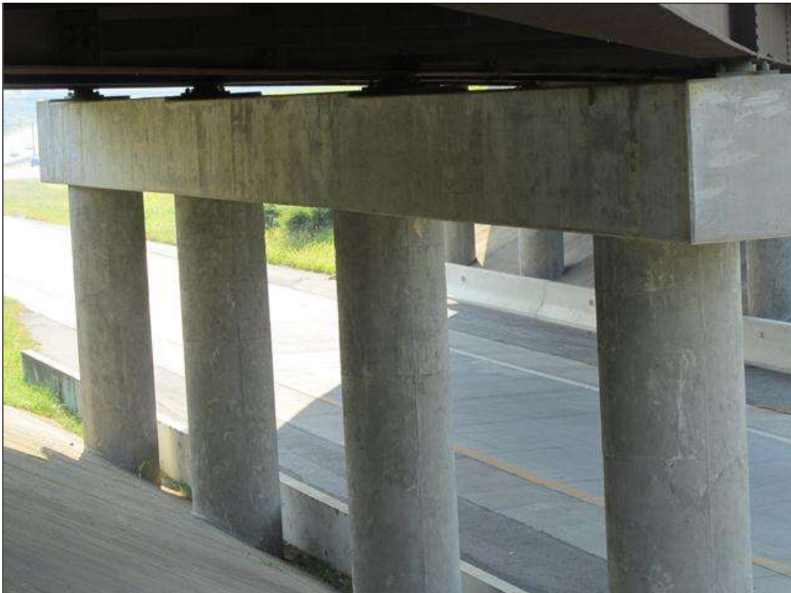
PIER 1 LOOKING NORTH
