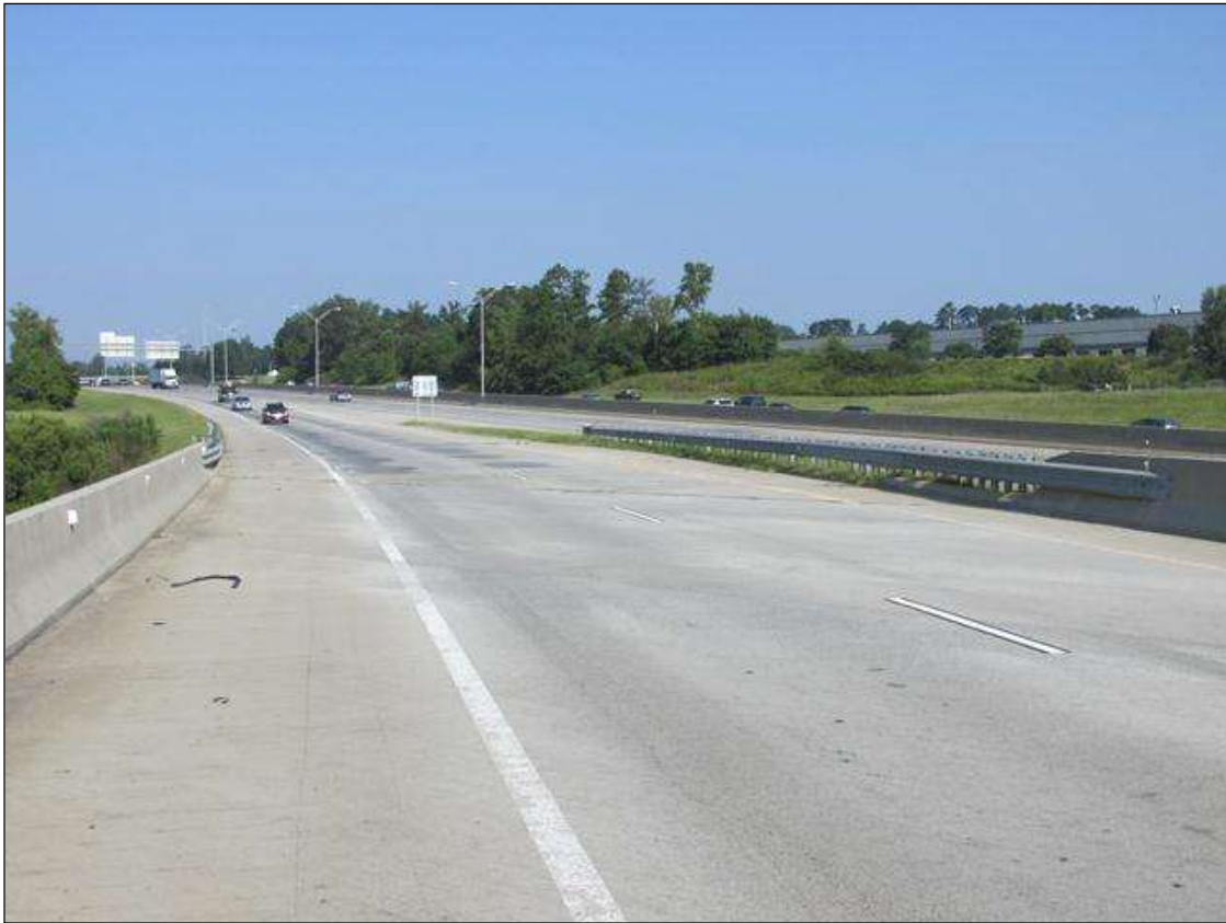
GUARD RAIL LOOKING SOUTH
