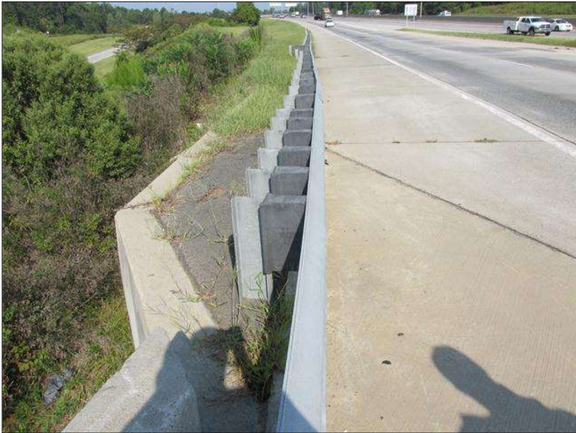
GUARD RAIL POST SPACING AT THE SE CORNER SW AND NW SIMILAR
