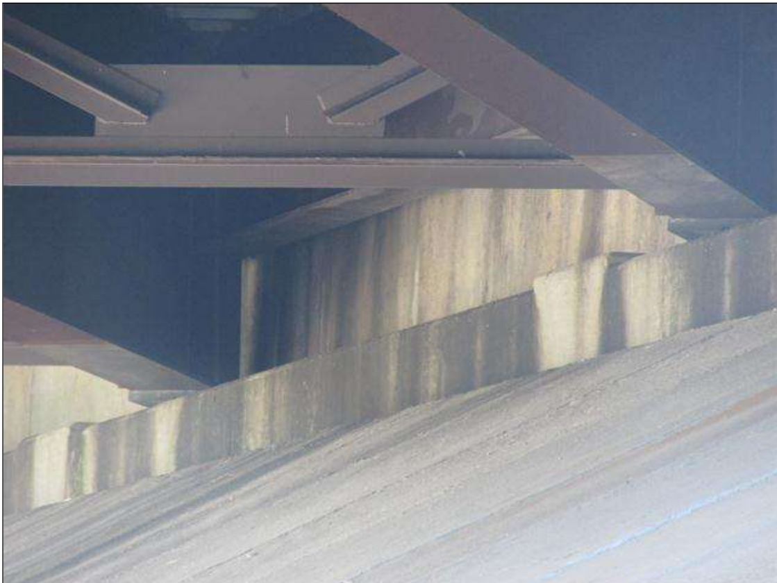
STAINS ON ABUT. 2 CAP DUE TO DAMAGED JOINT
