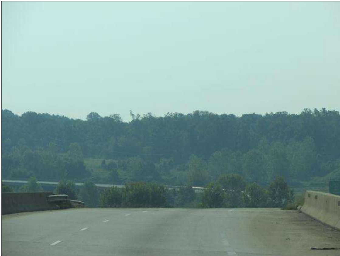
GUARD RAIL LOOKING NORTH
