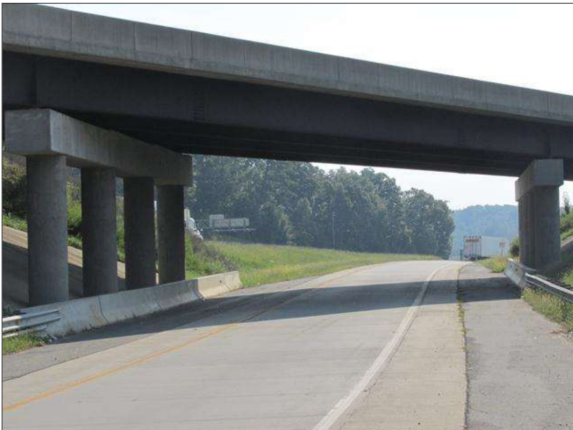
WEST OPENING, SPAN 2
