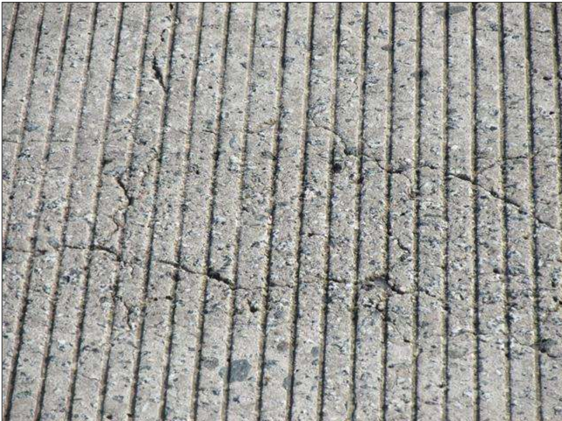
MAP CRACKS IN ALL SPANS UP TO 1/8" WIDE
