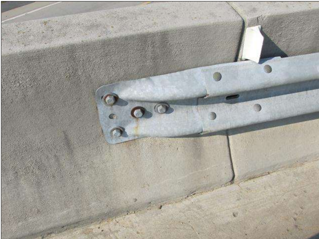
GUARD RAIL CONNECTION SE CORNER SW AND NW SIMILAR
