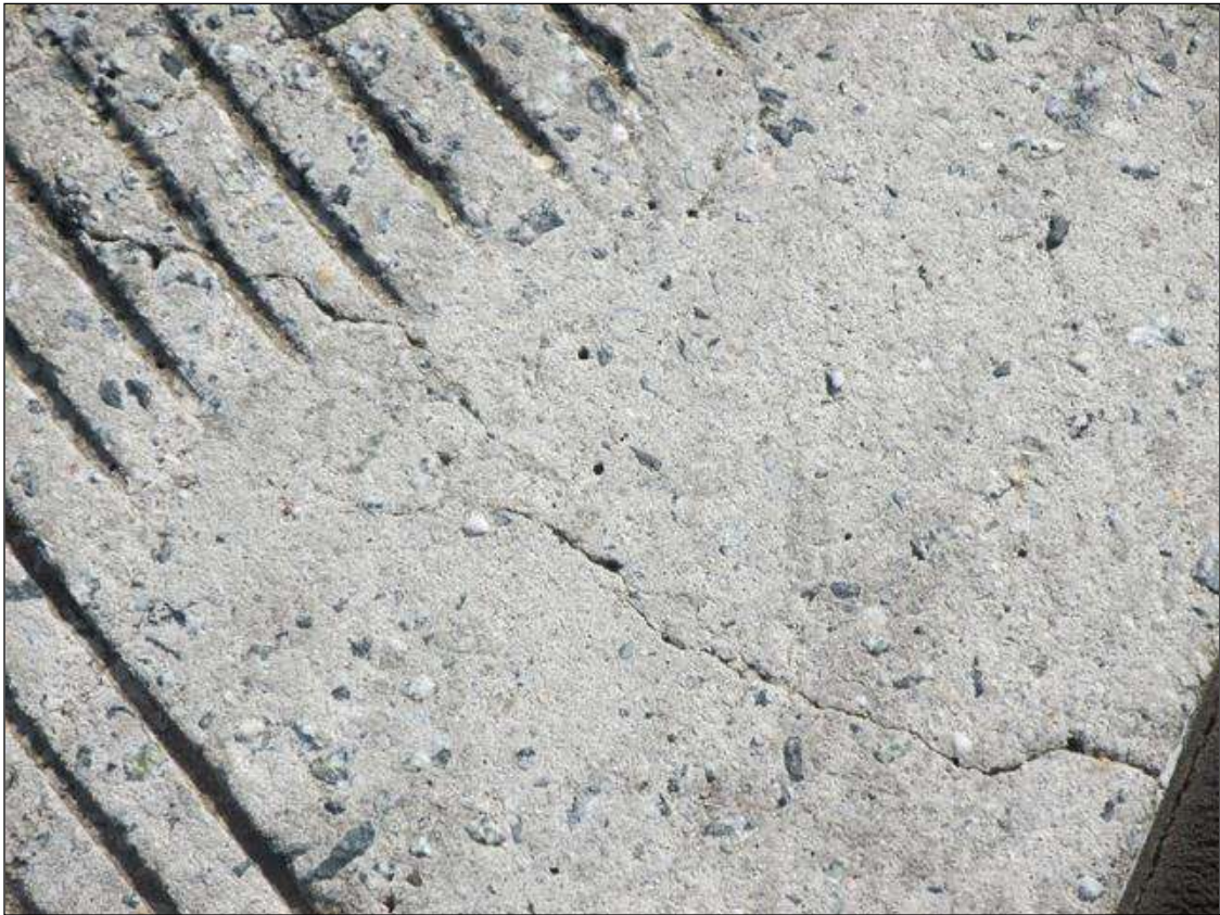
CRACKS IN THE SPAN ENDS
