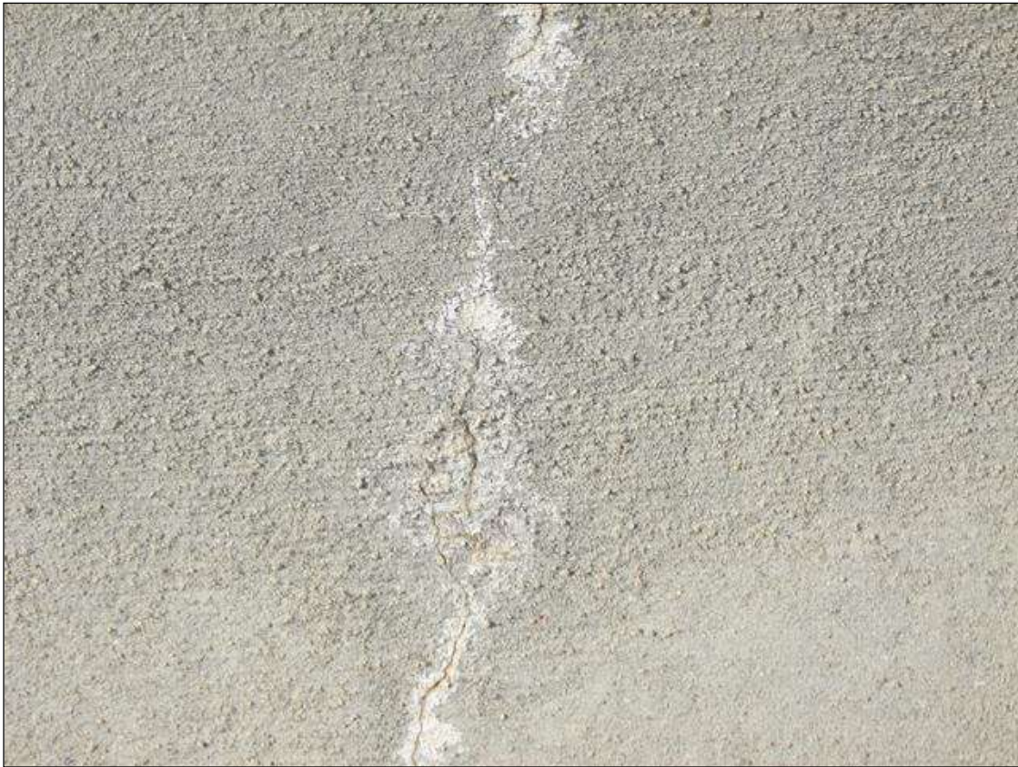
CRACKS IN BOTH RAILS
