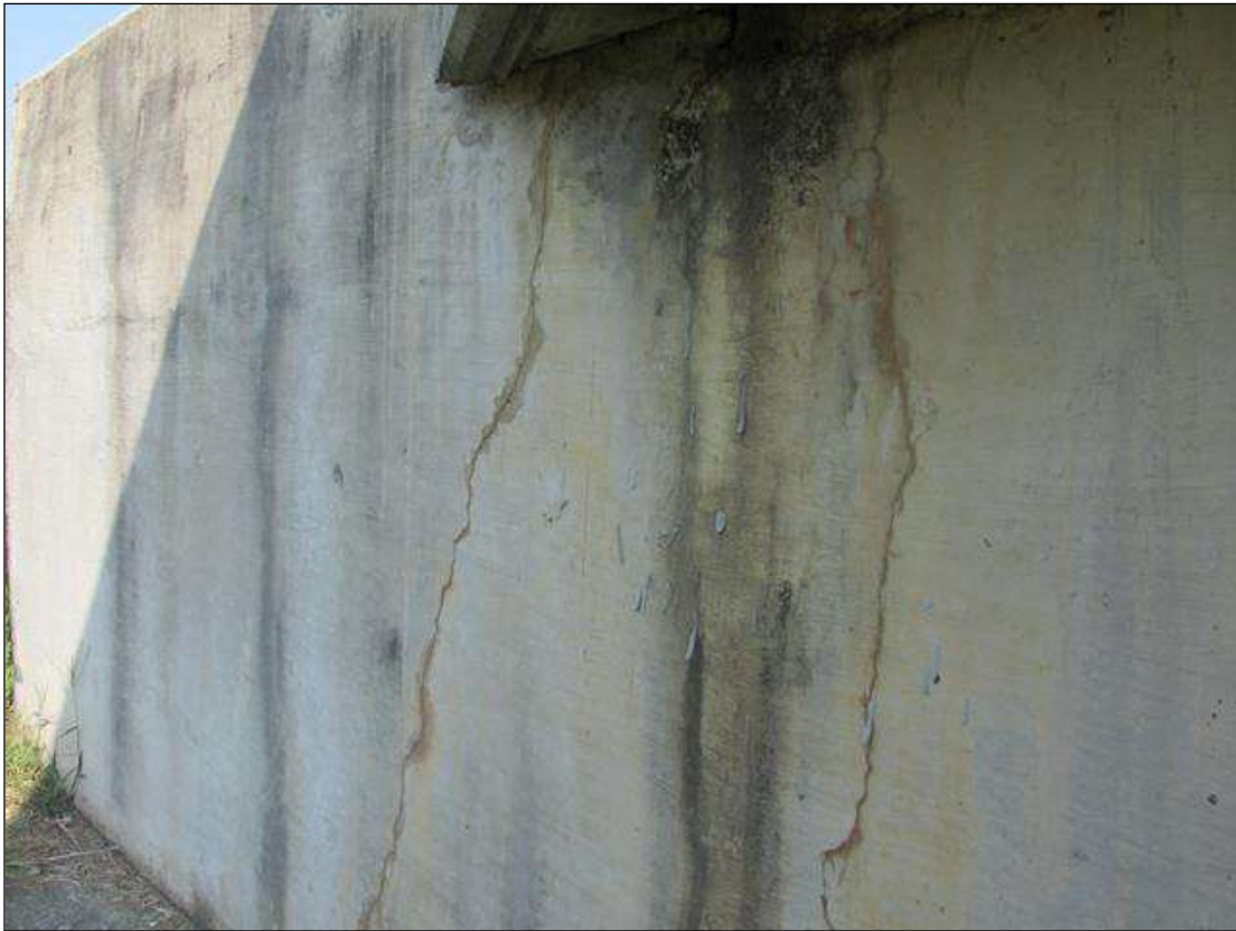
CRACKS IN BOTH ABUTMENT BACKWALLS
