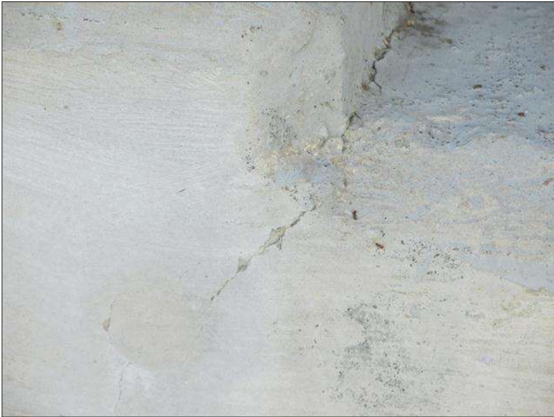
HL. DIAGONAL CRACKS IN ALL CAP STEPUPS
