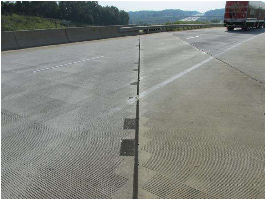
EXPANSION JOINTS AT BOTH ABUTMENTS
