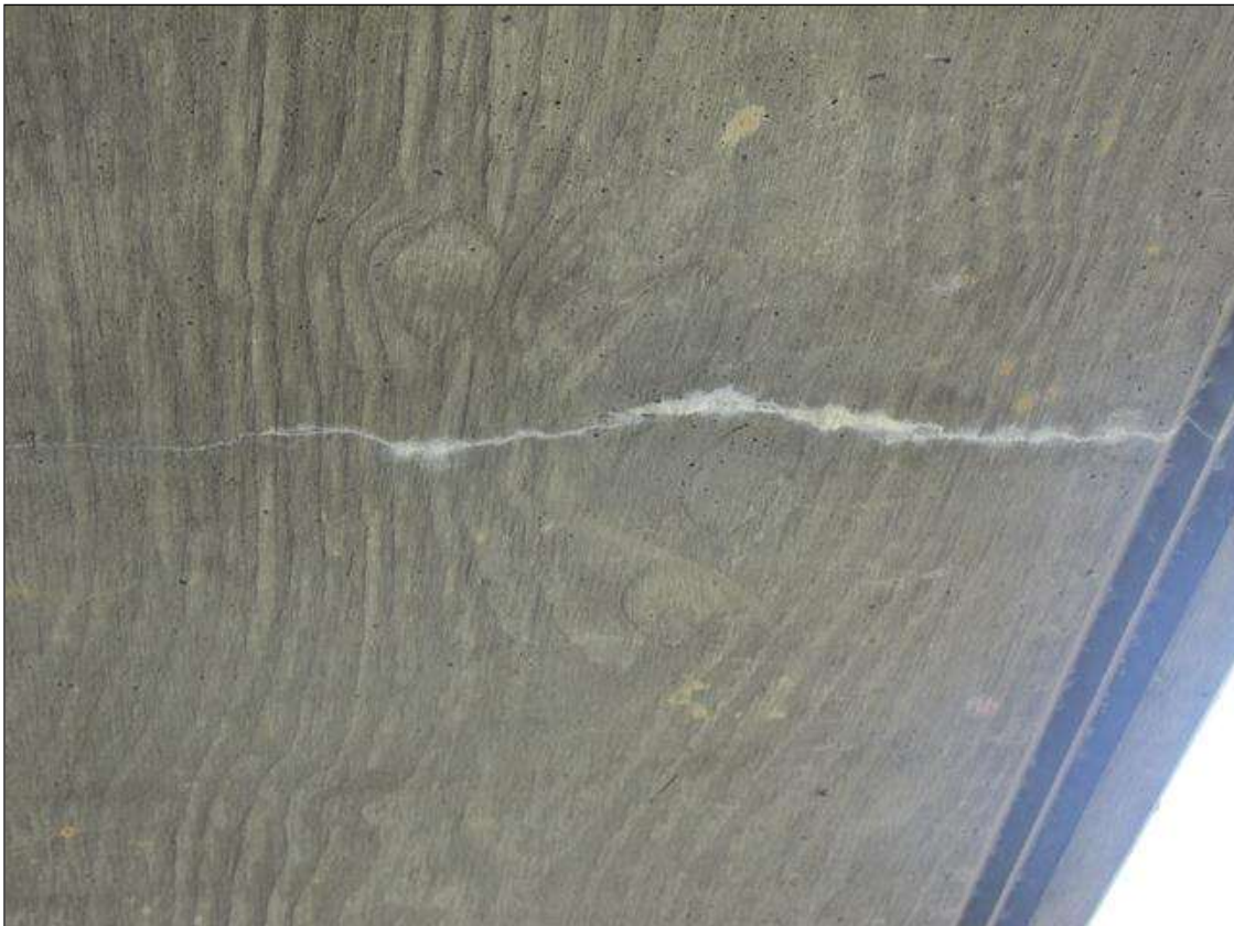
CRACKS IN BOTH OVERHANGS
