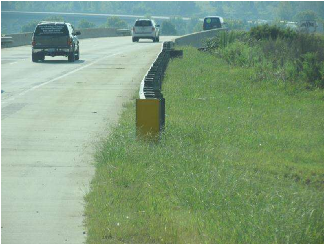
GUARD RAIL TERMINAL END AT THE SE END SW AND NW SIMILAR
